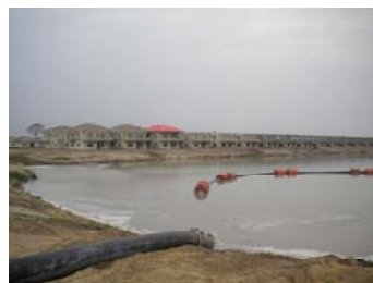
Row of Sirocco units by the Lake
