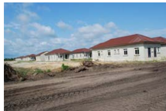
Sahara units at roofing level
